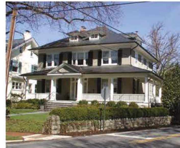
Chevy Chase Village- a Four-Square home featuring a centered front door with side lights. Hip roof with broad roof overhangs is typical of the architecture. Asymmetrical porch with pediment may have been remodeled. Paired double-hung windows are commonly seen in this style. Pebble-dash stucco looks to be original.
