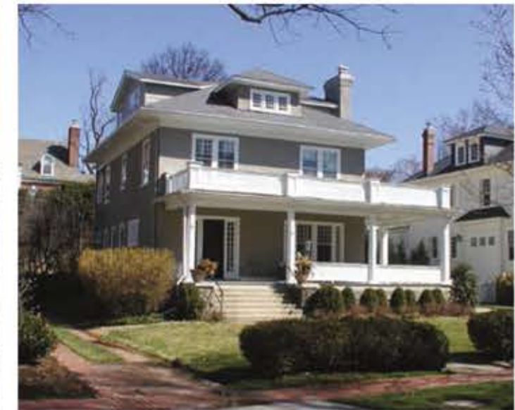
Chevy Chase Village- a Four-Square home with side entrance, asymmetrical porch and windows grouped in pairs. The dormer in the front appears to be original while the side dormers appear to be additions. Pebble-dash stucco was used throughout.
