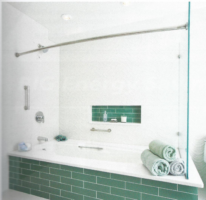
Photo by Geoffrey Hodgdon. This Wentworth bathroom includes a tub with built-in niches and an unobtrusive grab bar for safety and ease.
