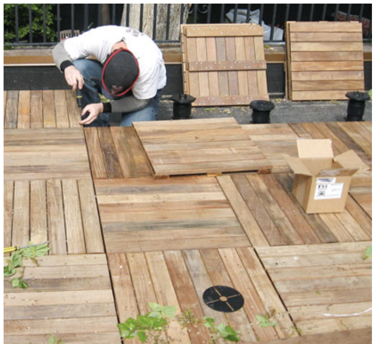
Figure 4. A plastic disk and a single screw secure the corners of four ipe tiles at every pedestal (above). Spacer tabs maintain a uniform 1/4 -inch gap between adjacent tiles; a wedge-shaped cutout in the disk can be rotated to allow a tile to be removed. Tiles and pedestals are installed and leveled one at a time (right).
