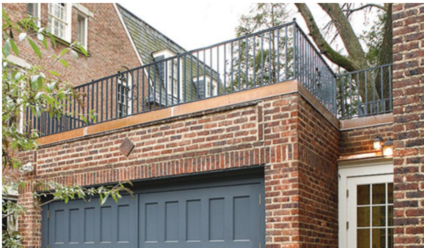
Figure 2. New copper flashing fitted around an iron deck railing serves as a waterproof cap over the parapet.
