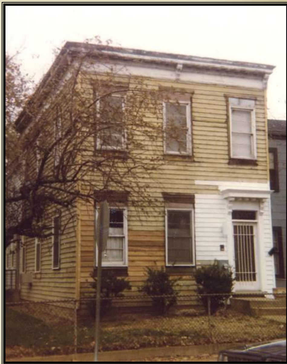
During Façade Restoration
